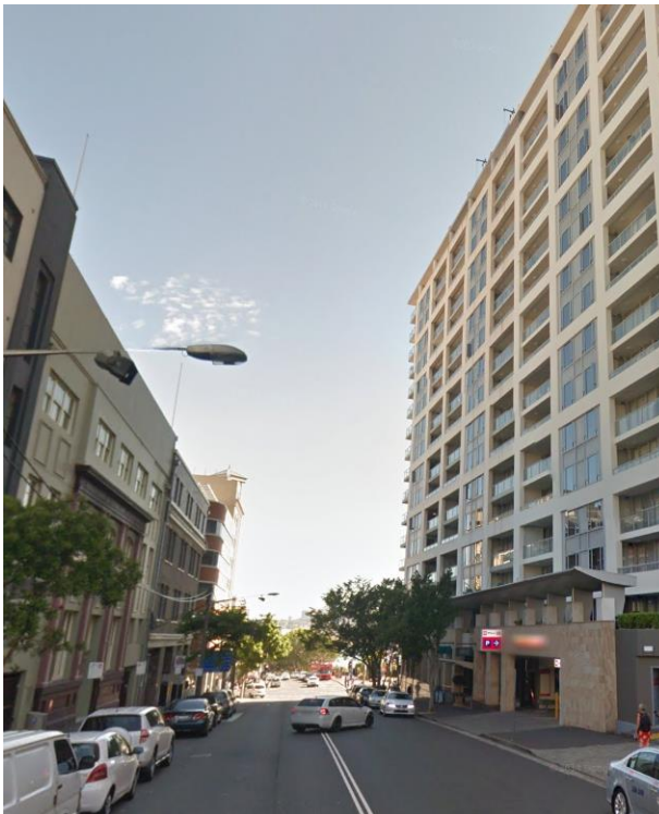
PICTURE 5 – 50 MURRAY STREET LOOKING NORTH
