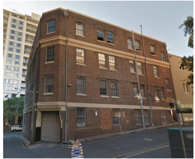
PICTURE 4 – 47 MURRAY STREET LOOKING EAST
